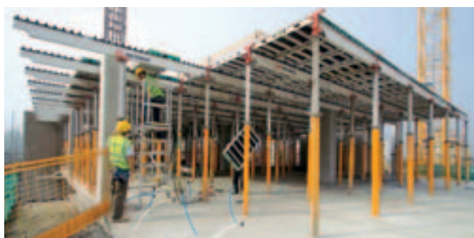
SKYDECK: Safe erection from below does not come at the cost of a high quality finish.
