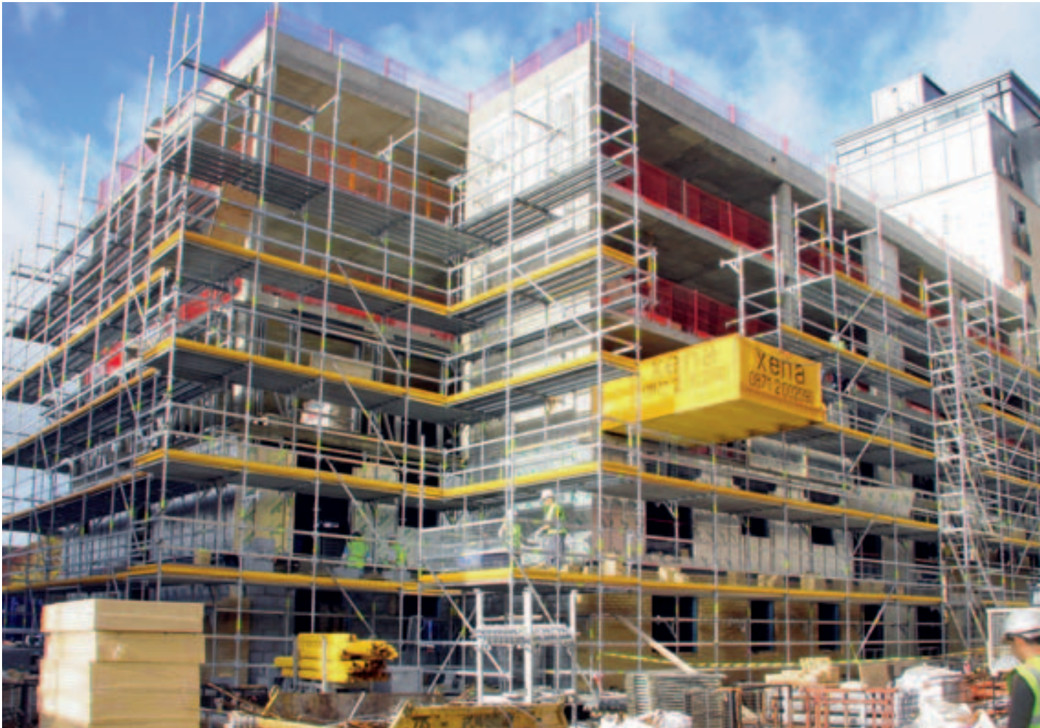
PERI UP Industrial façade scaffolding.
