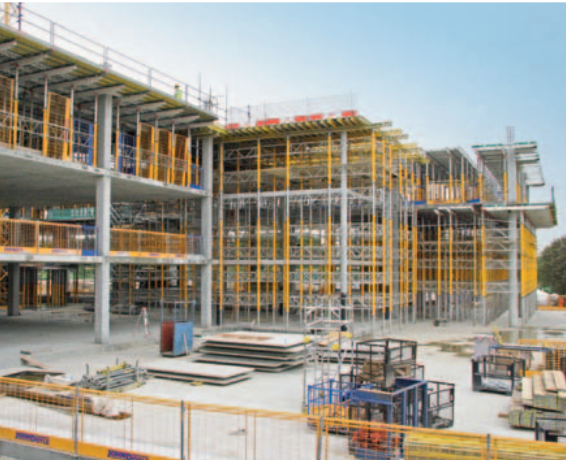
11.50 m high falsework supports the soffit of the central atrium.
