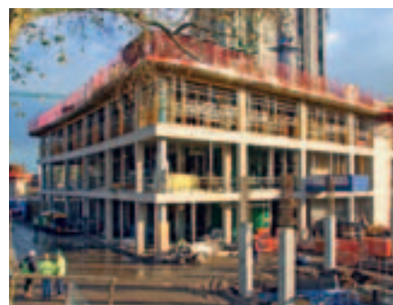
SKYDECK and MULTIPROP used to form floor slabs.
