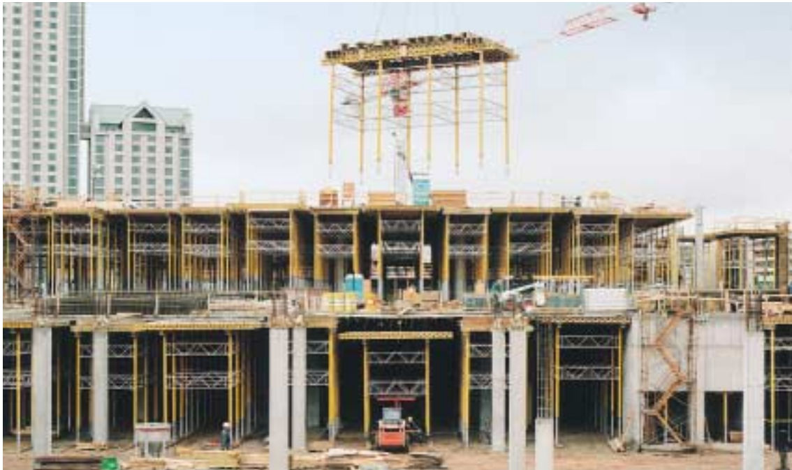
Large MULTIFLEX tables flown easily and safely.
