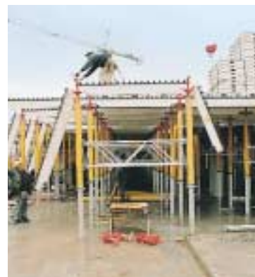
The patented main beam design allows a crew of two men to easily erect the SKYDECK system.
