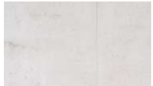
High quality finish with VKS: Minimized offset between panels.
