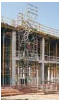
The PERI UP stair tower provides safe and easy access.
