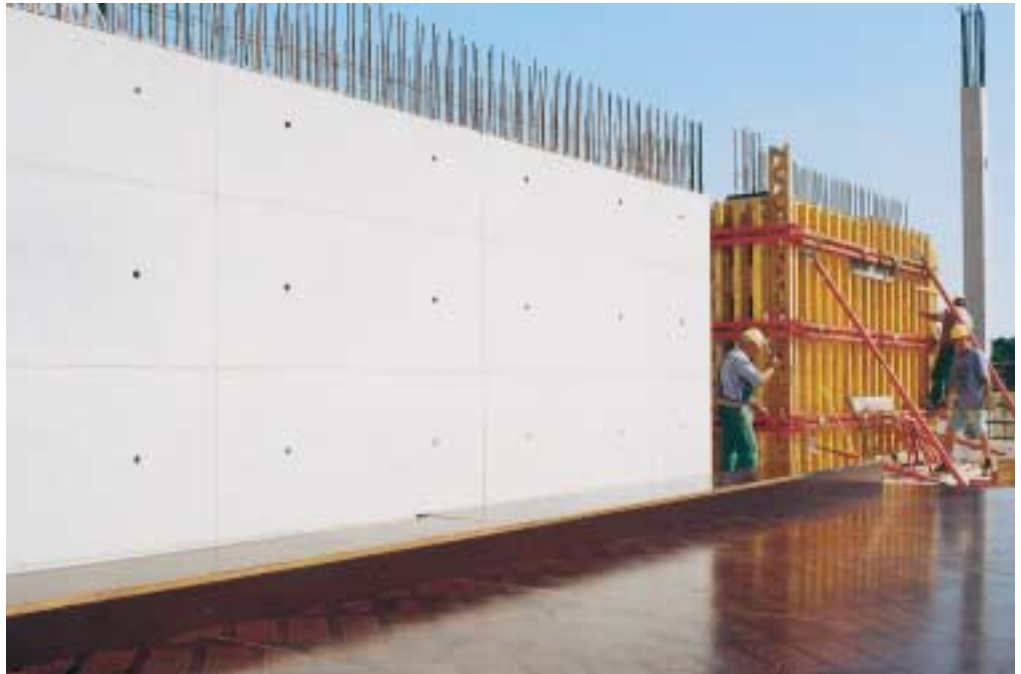
Perfect architectural concrete with horizontal and vertical pattern.
