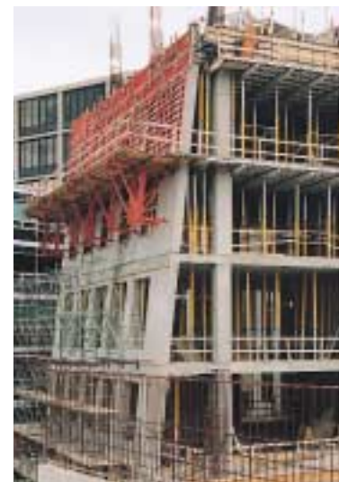
TRIO Wall Formwork in conjunction with PERI's KG 240 climbing brackets met the requirements of forming the 10° sloped walls.
