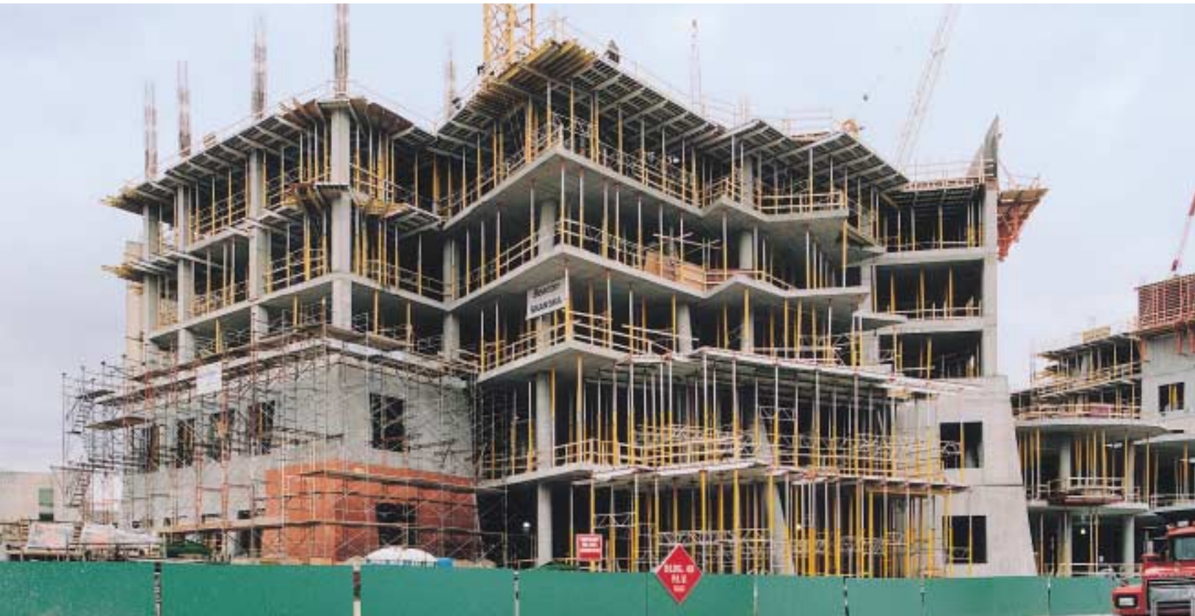
Cantilevered slabs with continuous shoring using the MULTIPROP.
