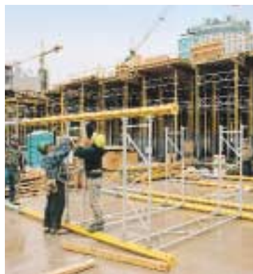
Large MULTIFLEX tables can be erected from the ground with minimal effort.
