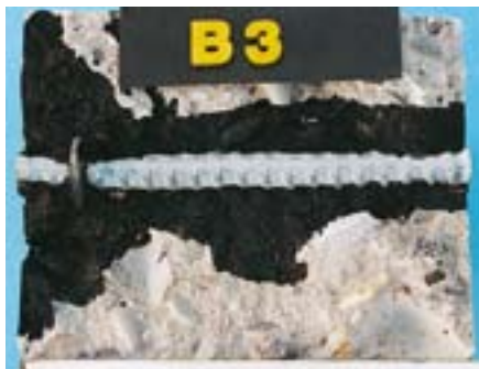
Formation of shrinkage cracks makes tie rods...
